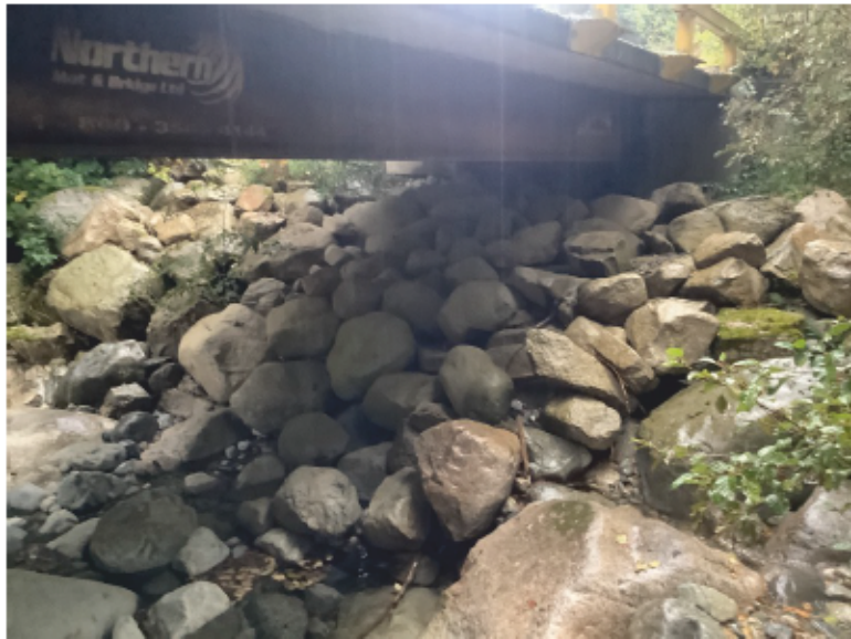
Right Bank Abutment when facing downstream
