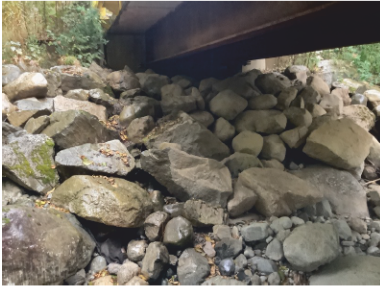
Left Bank Abutment when facing downstream
