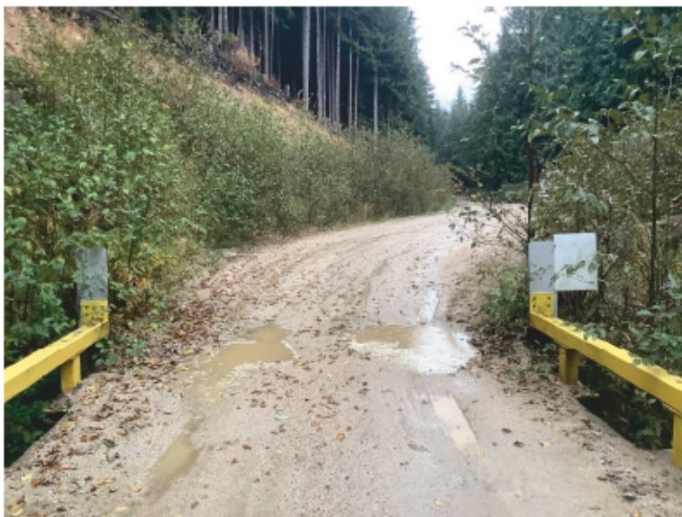
Approach from bridge deck of Left bank approach when facing downstream
